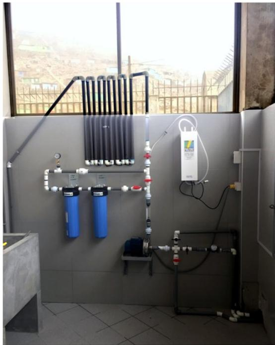
*The water filtration system on the front wall of the new water room at Reimagine headquarters*
